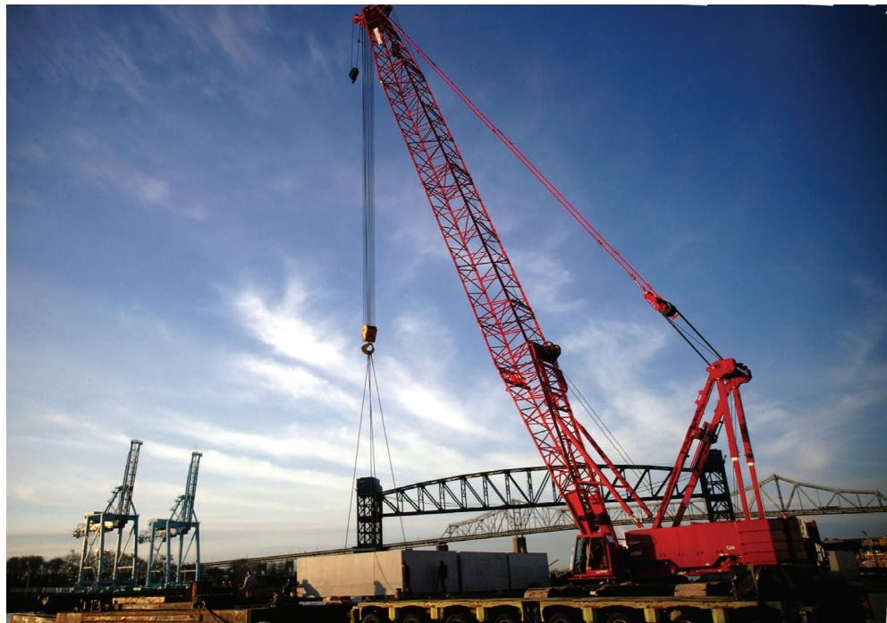
**Description:** CME crew placing a 160,000 pound pre-cast concrete form on to a barge. This unit is one of 6 for this shipment with 15 scheduled for delivery totaling 2,400,000 pounds.
